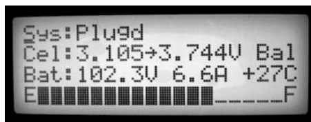
Figure 5.67 Graphic screen for the Lithiumind BMS.
